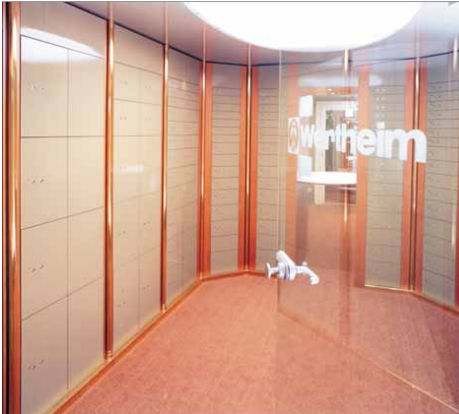
Electronically controlled safe deposit boxes in vault EET 070
